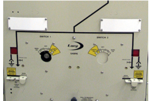
Ring switch mechanism
