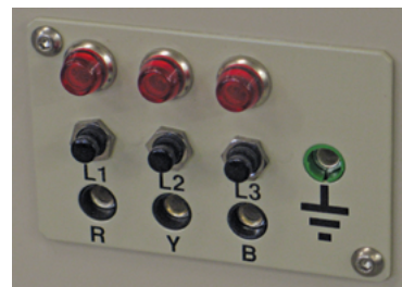
Neon indicator with push-to-test buttons
